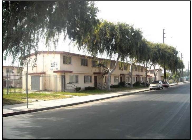
View of Jordan Downs residences along Grape Street.
