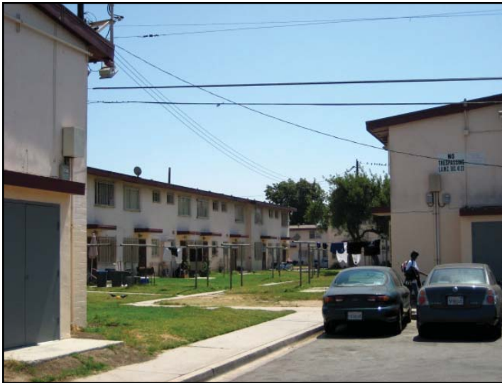
View of the rear entrances of Jordan Downs residences and parking area.
