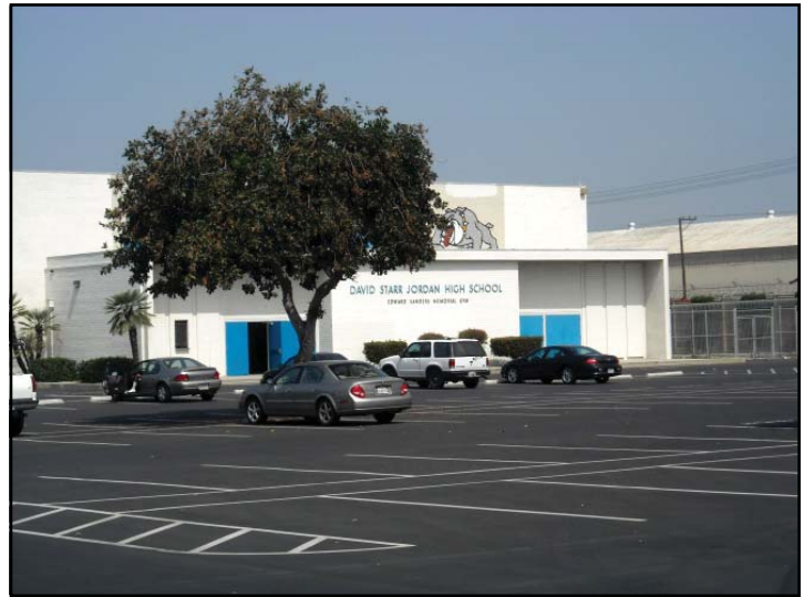
View of the LAUSD-owned property from Alameda Street.
